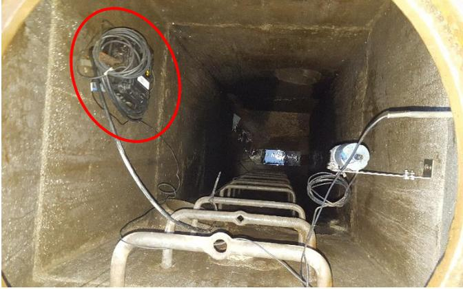
Figure 2-25: Installation of the Battery Pack of Flowmeter at the Outfall of the Studied Sector
