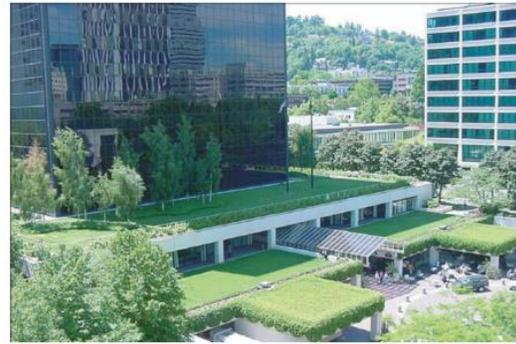
Figure 1-5: Vegetated roof (Fuamba et al. 2010)
