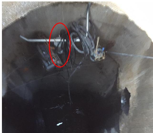
Figure 2-34: Installation of the Data Logger of the Turbidity Meter
