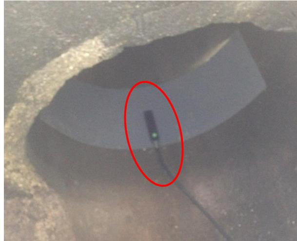
*Figure 2-30: Installation of the Flowmeter Probe at the Main Collector Pipe Downstream the Retention Tank*
