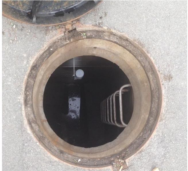
Figure 2-20: Water Depth Meter installed in the Retention Basin of the Studied Sector
