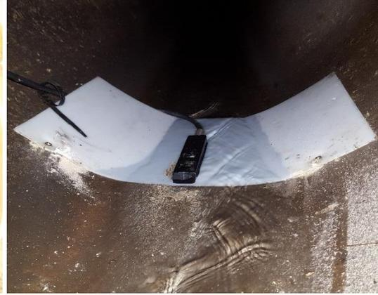
Figure 2-26: Installation of the Flowmeter Probe at the Pipe Existing the Outfall of the Studied Sector
