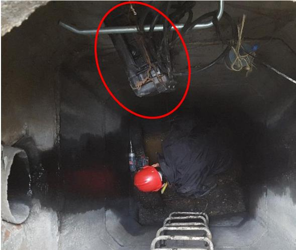
*Figure 2-29: Installation of the Battery Pack of Flowmeter Downstream the Retention Tank*
