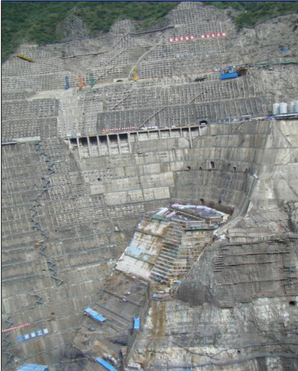
*Figure 5.2 The height steep rock slope during the phase of excavation*
