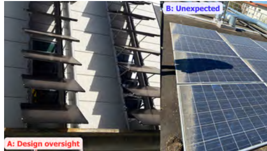
Figure 3: Some example of unexpected shadows. A is mostly a design oversight, while B is unexpected build-ups.
