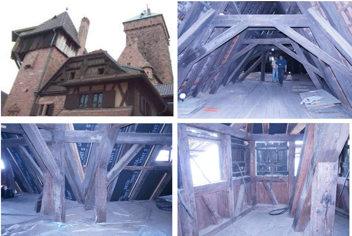
Figure 3.26. Castle of Haut-Kœnigsbourg (top left) and details of its truss structure (top right and bottom).
