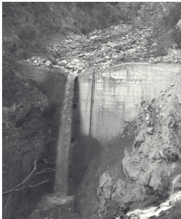
Figure 1.4 – The 34-m-high ‘Fèvre’ check dam in the Bonrieu branch of the Saint Martin torrent (73 - FRA.); 4-m-thick at the crest, 7.6-m-thick at the toe, construction: 1939-1942, just upstream of the huge lateral Bon Rieu landslide (Messines du Sourbier, 1939a). The downstream gorge is currently filled by the landslide movement, stabilizing it. The dam is still in good condition, almost completely buried by the landslide, and it fulfills its function perfectly: decrease the energy and erosive power of debris flows upstream of a reach whose incision has catastrophic consequences (photo Apr. 1955 by L. Anchierri courtesy of RTM73).
