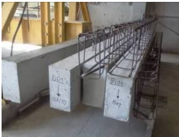
Figure IV-13. Steel cages and mould used for beams
