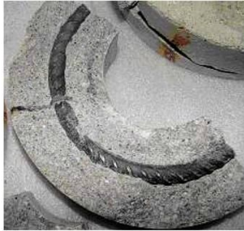
Fig.III-27. Uncracked sample kept for 500 days in a wetting-drying in saline environment: no corrosion or no corrosion crack [22]
