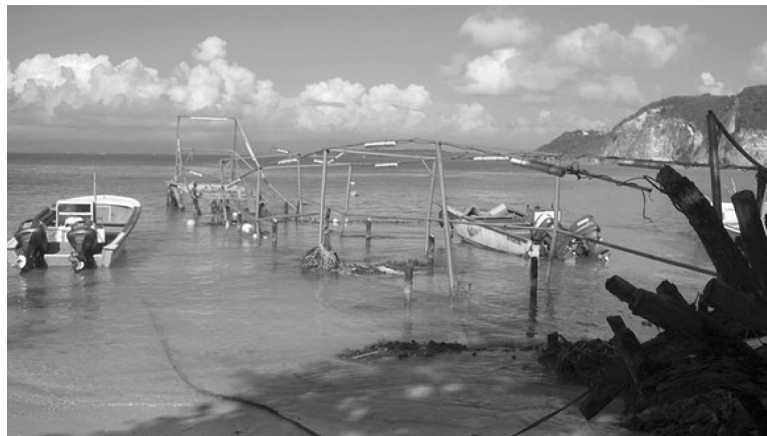
Fig. 10 Destroyed berth in Petit Havre
