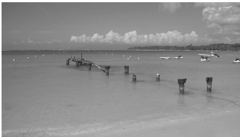
Fig. 15 Destroyed berth, Sainte-Anne
